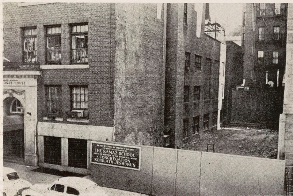
Before long, the new building will rise on this site
