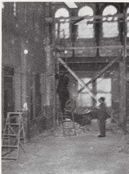
The Social Hall being prepared for a "face lifting" which will change it to a modern up-to-date banquet hall.
